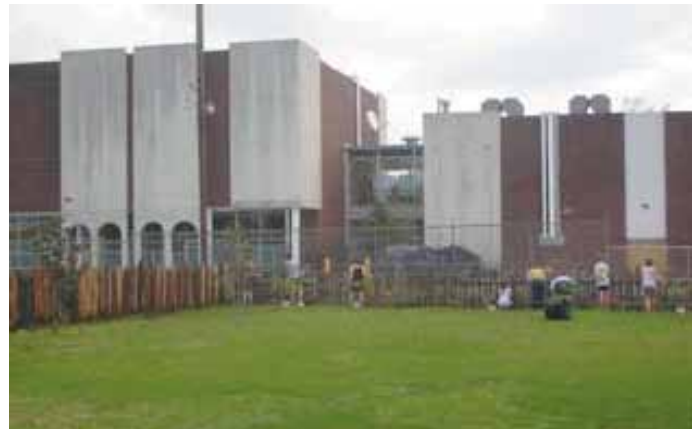
ABOVE: In this photo, the rear fence has been cleaned and is ready for the limewash application by the Tulane Preservation Technology students. Over the course of the semester, the students as a class and service learning student Gillian Faircloth returned several times to add coats of limewash to the rear fence. Photo by G. Faircloth.
