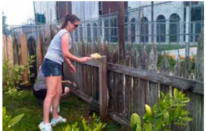
ABOVE: Tulane MPS student Kaylee Smith helps the rest of the 2011 Tulane Preservation Technology class add a coat of limewash to the Cabrini alleyway pieux fence.
